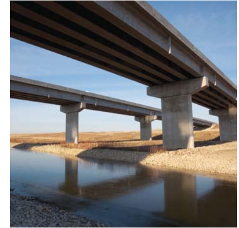
Winnipeg floodway, Winnipeg, Manitoba Richard Gillard
