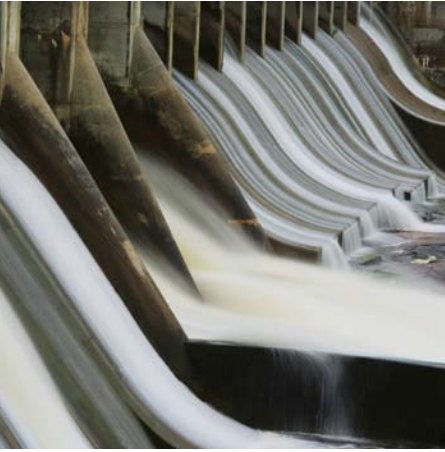
Hydroelectric dam, Manitoba Ian Graham
