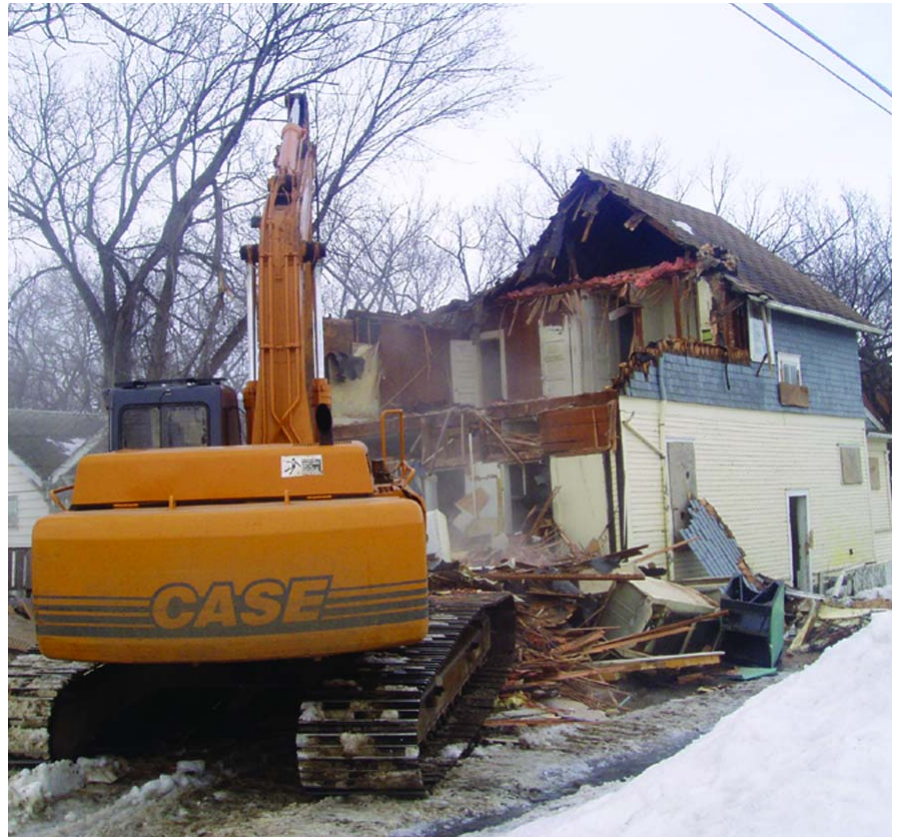
Some substandard houses are being demolished, making room for new construction
