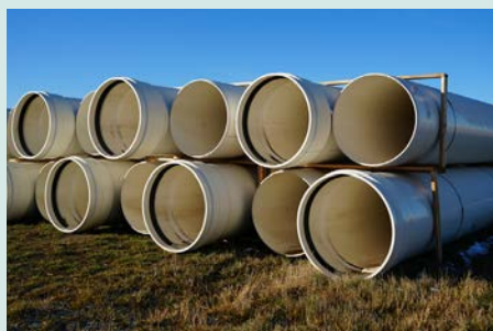
Irrigation pipes at a construction site near Chin, Alta. (Photo courtesy of CIB)
